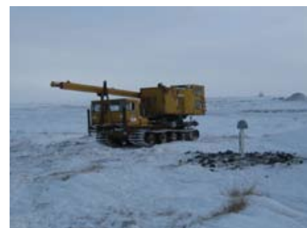
The completed permafrost monument with the drill rig in the background.
