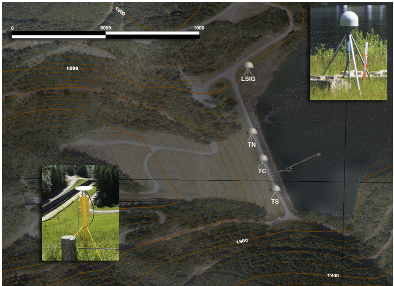
Fig. 4. (Color) Aerial view of the earth-filled Tolt Dam, with three GPS stations installed along its crest and a fourth one used as a reference station (LSIG) located on bedrock (Imagery © 2015 Google, Landsat, USDA Farm Service Agency, Map data; inset images by Rex M. Flake)
